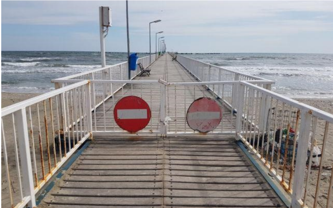
Image of metal footbridge in Mamaia source Adevărul newspaper
