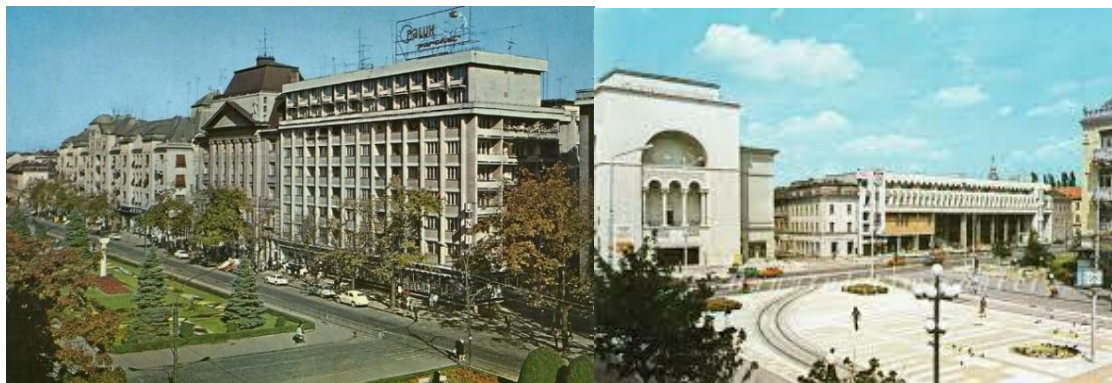
Fig. 8: (left) the blocks on the east front. Fig. 9: (right) north front (Opera and Modex building)
