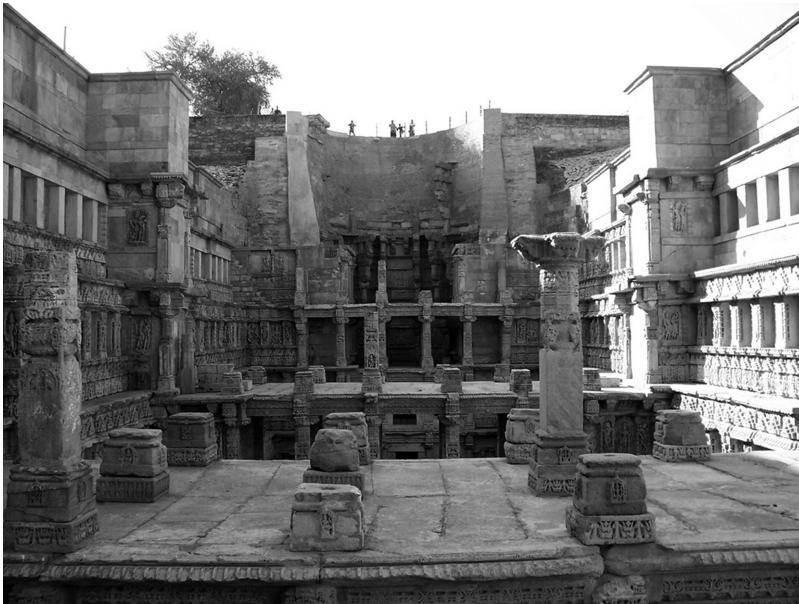
FIGURE 7.3 View of stepped corridor from east
