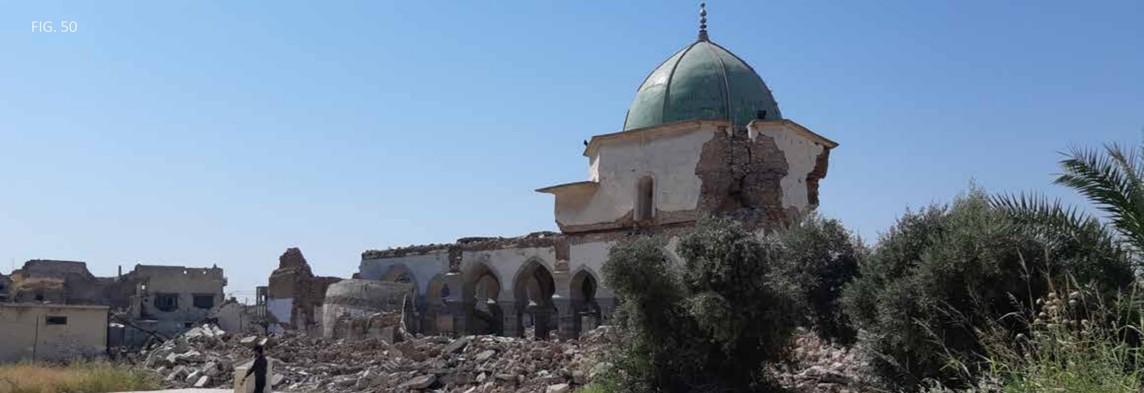
Situation in 1438 AH / 2017 AD after the intentional destruction (Figure 50 and 51)
